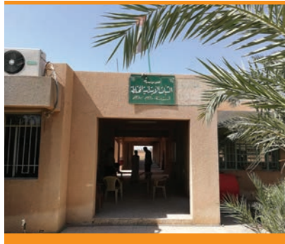
Agility - Iraq renovates washroom facilities and outfits classrooms for a girls' school in Basra that enrolls 500 students a semester.
